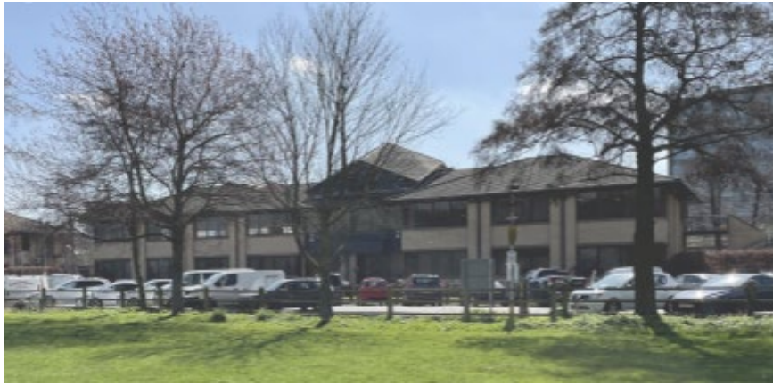
Figure 2 - photographs – front of existing office building viewed from Kings Meadow from the opposite side of Napier Road
