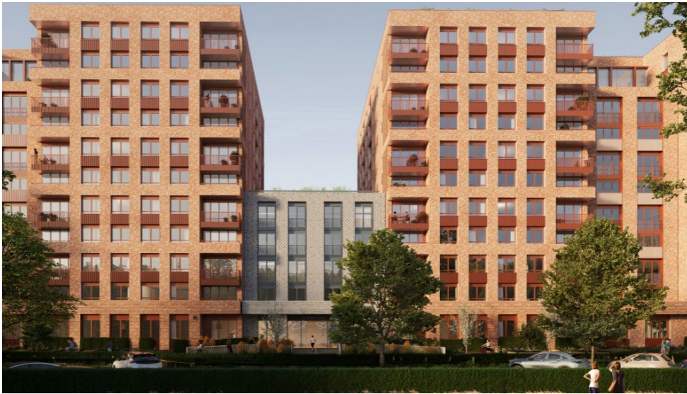
Figure 5 – Five storey high link blocks
