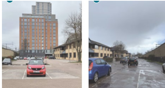
Figure 18 – Existing view looking west and east from the rear car park showing the Network Rail retaining wall
