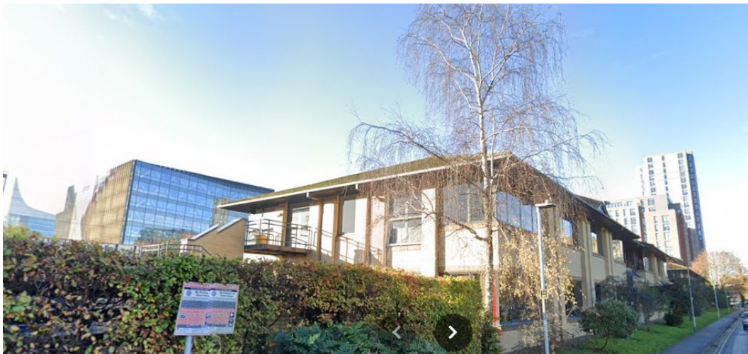
Figure 29 – Existing view looking west along Napier Road
